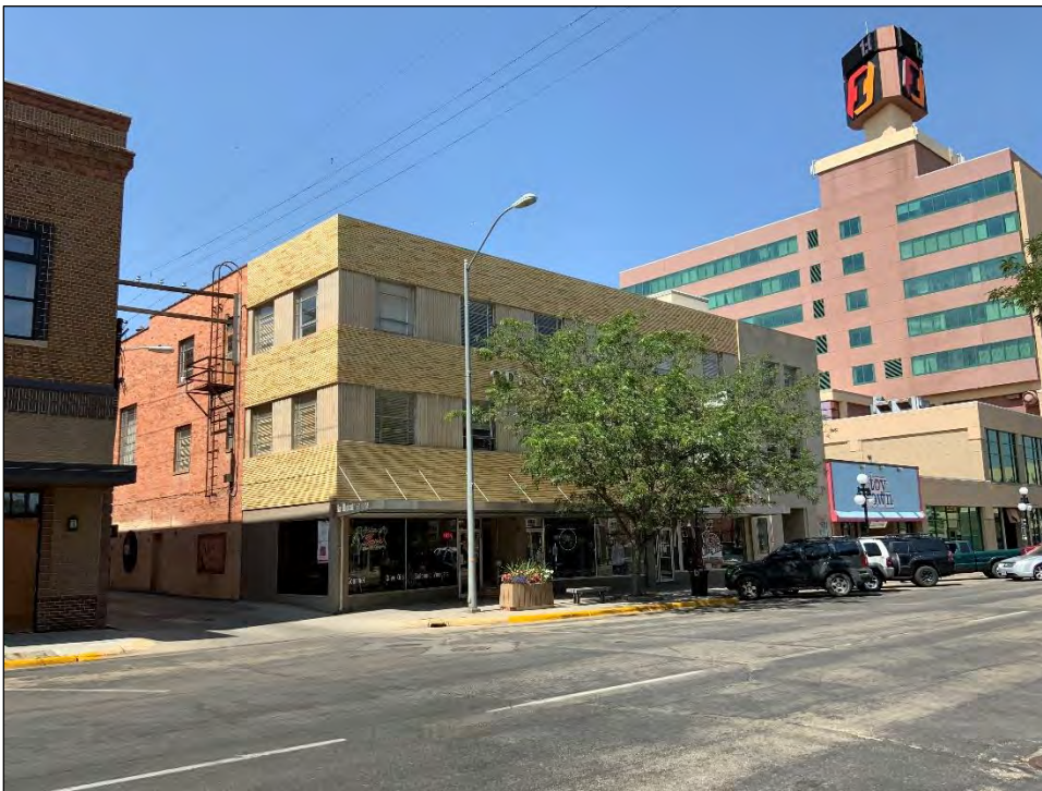
Photo 15. Overview image of the Odd Fellow's building in downtown Casper, view northwest.
