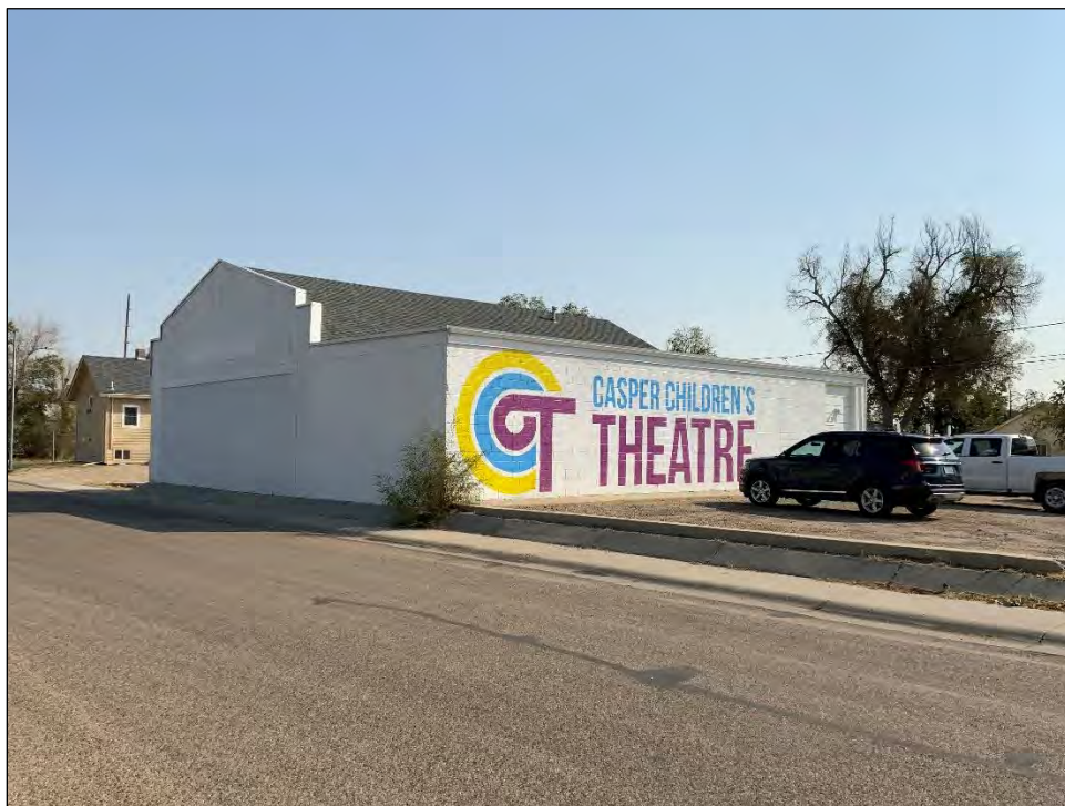
Photo 21. Overview image of the Second Baptist Church now the Casper Children's Theater, view northeast.
