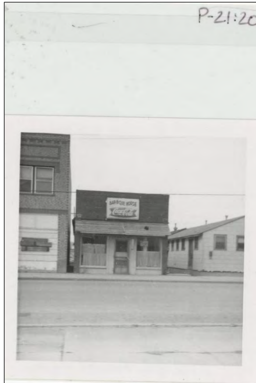
Photo 3. Representative image of a false front store (center) as well as brick construction (left) and tarpaper/shingling (right). Image courtesy of the Western History Center.
