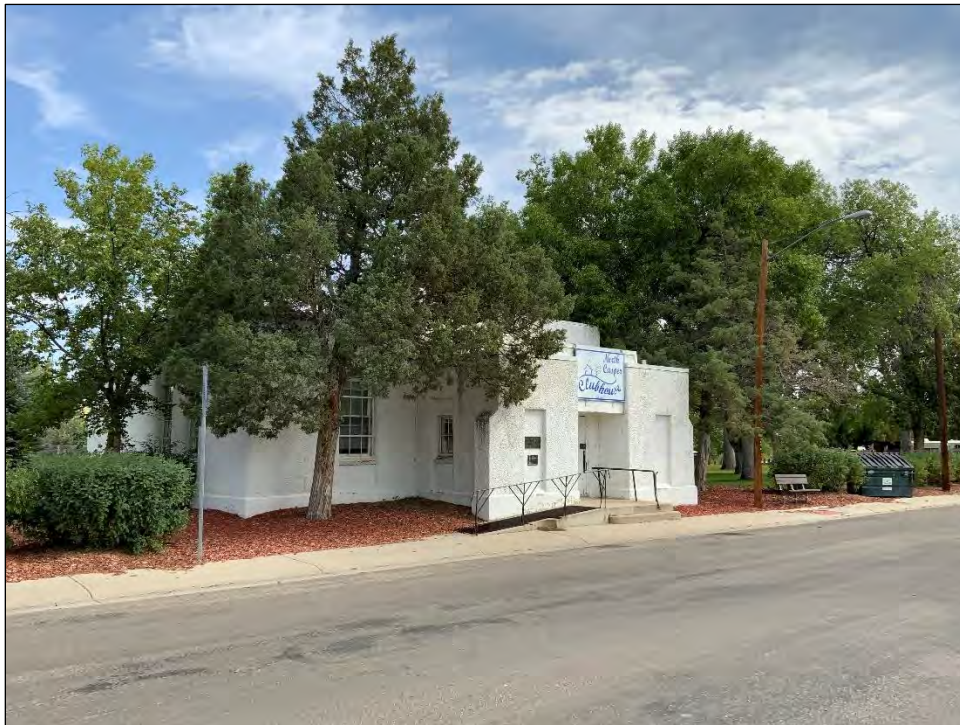
Photo 10. Overview image of the North Casper Clubhouse view north-northeast.
