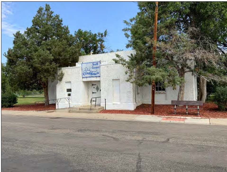
Photo 8. Overview image of the North Casper Clubhouse view north-northeast.
